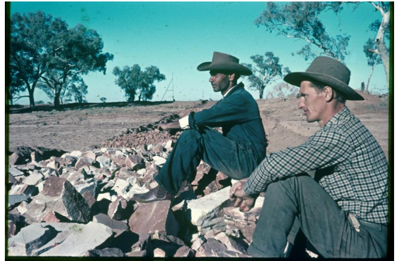
Work on the Stuart Highway (south of Alice) [Northern Territory Public Works Department]
